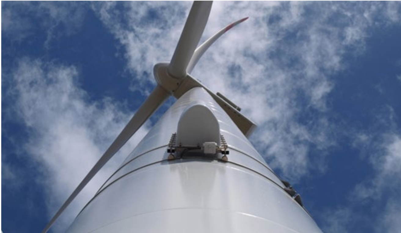
WEA Turm Installation
